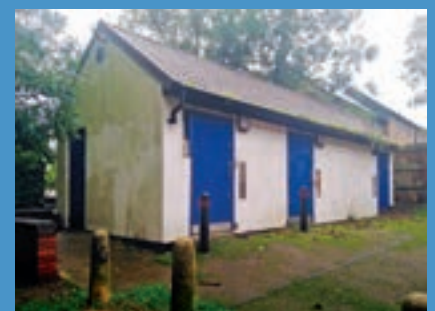
The current state of the disused toilet building in Dronken Lane
